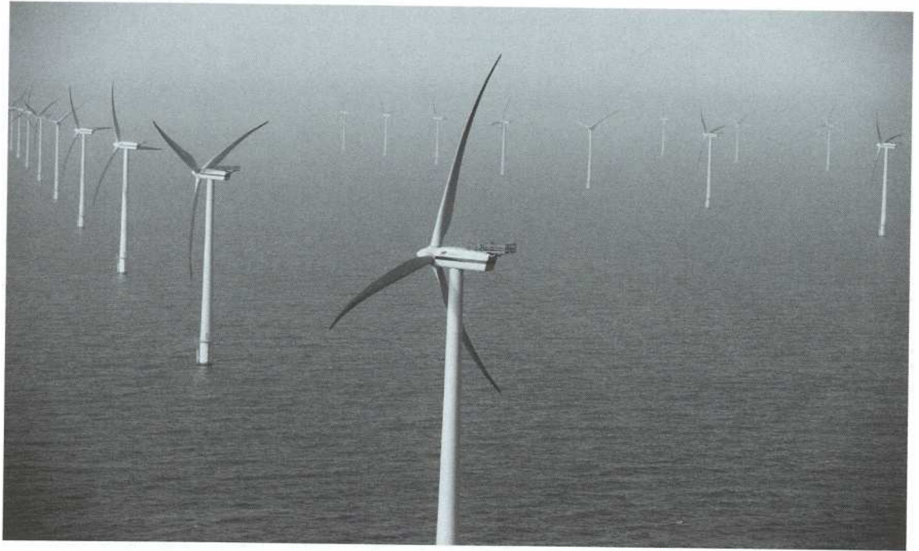
Figure 13.2 Large wind turbines on a wind farm off the coast of Norway. Notice the large amount of bending on the blades, suggesting that they are operating at high thrust and generating maximum power. Source: Photo courtesy of Sandia National Laboratories.
